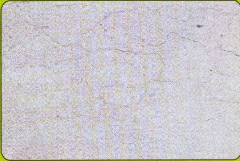
Picture of road laid without plastic compounds
